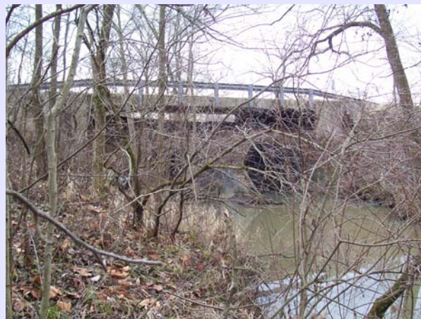
Blackford County Bridge 96
