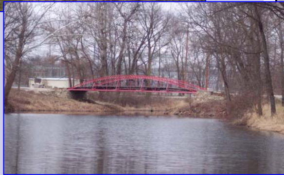
Canal era Transportation Enhancement project Delphi, Indiana
