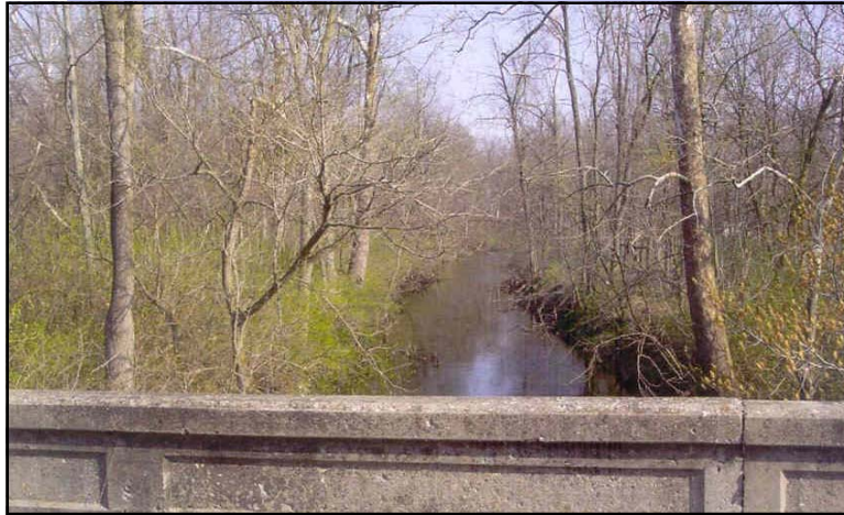
Tipton County Bridge 93 Replacement
